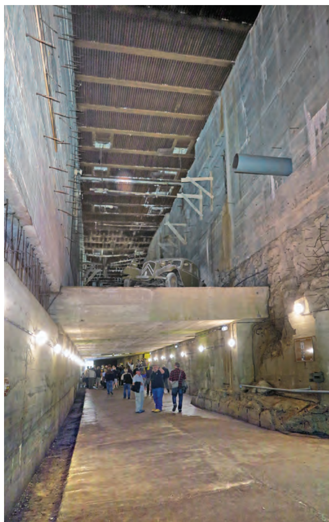
Inside the blockhouse servicing hall, North wall at L, wall of the LOx plant to R, walking where locomotives were to shuffle rockets through the stages of preparation.
